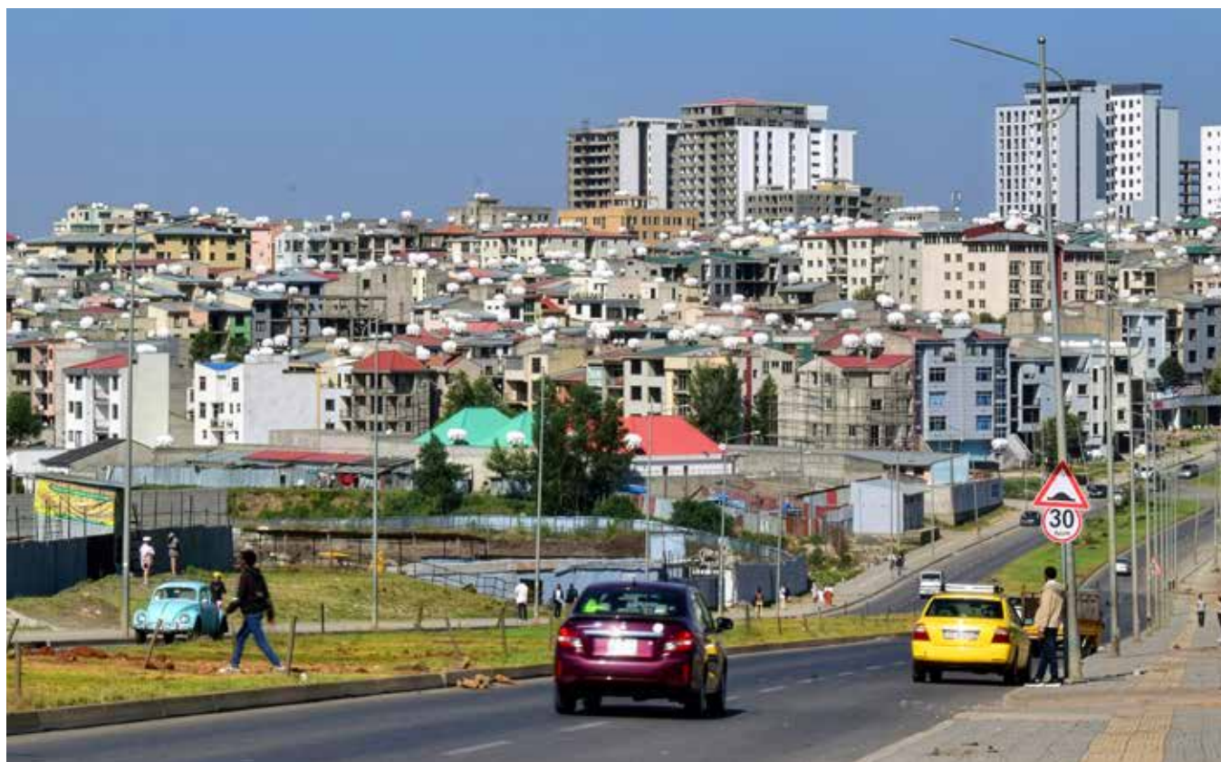
FIGURE 7 | Water tanks across Addis Ababa's buildings help residents circumvent poor water supply and meet the rising demand of the city's growing population
