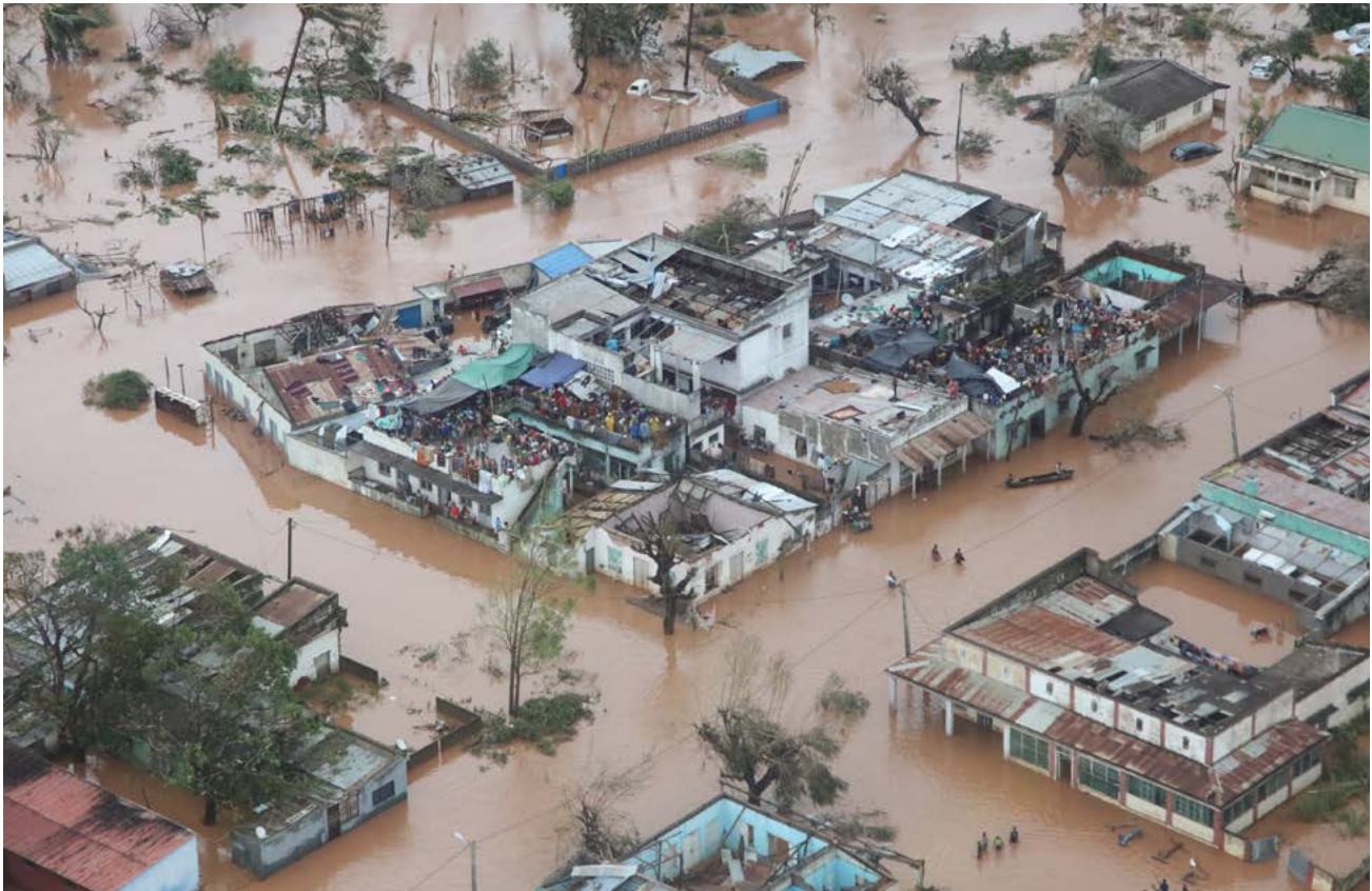
Residents taking refuge on rooftops in Mozambique during Cyclone Idai.
